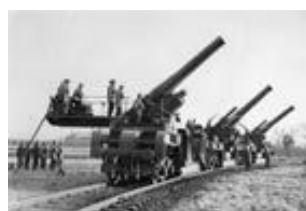
Railway howitzer 1916 12 inch gun range: 12,000 metres
